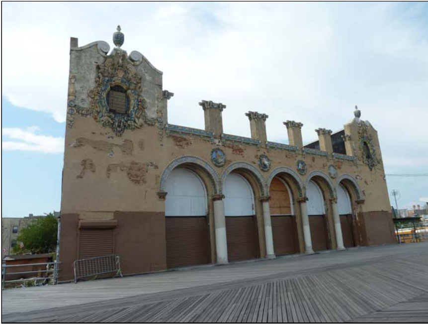
1. Southern facade fronting the Riegelmann Boardwalk.
