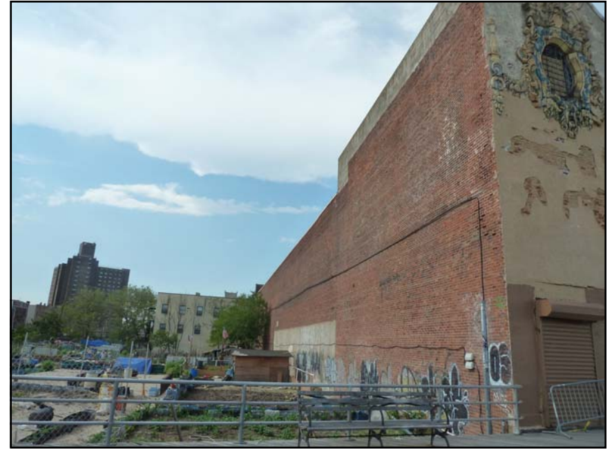
4. Western facade and adjacent decommissioned community garden.
