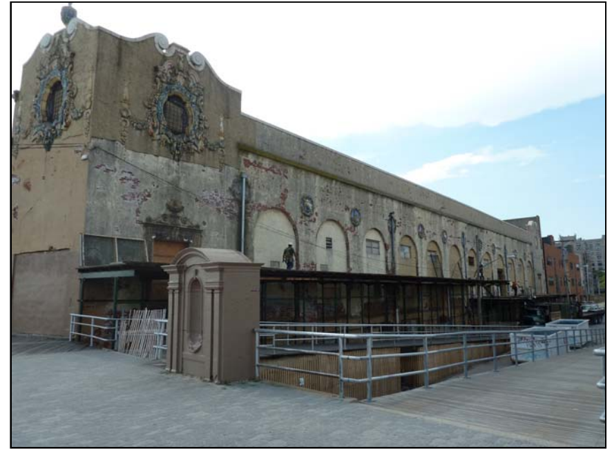
2. Eastern facade fronting West 21st Street.
