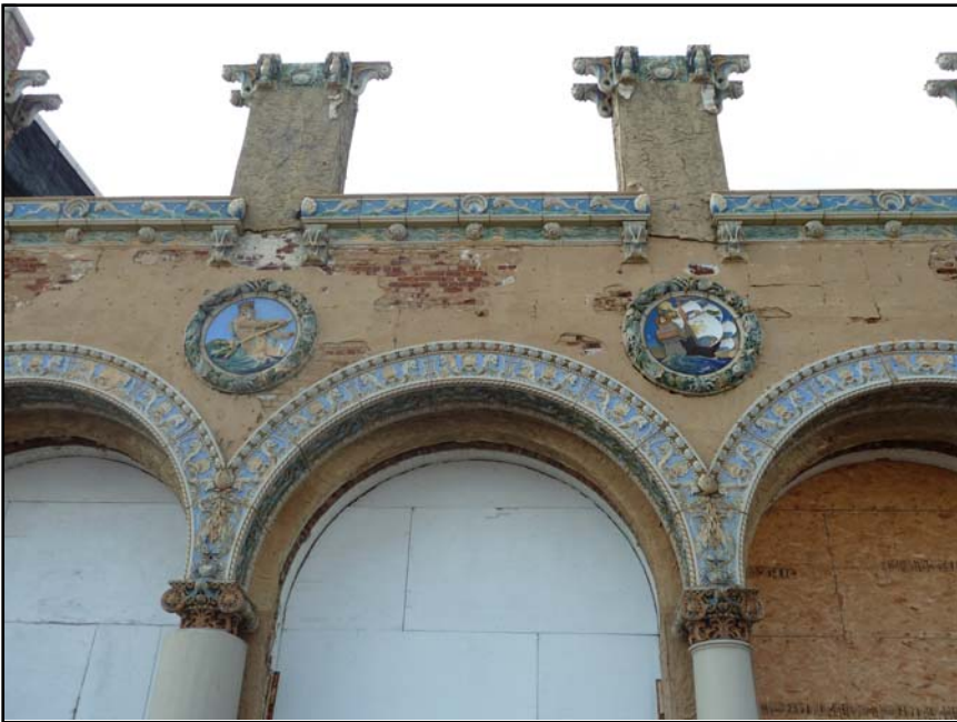
3. Southern facade details.
